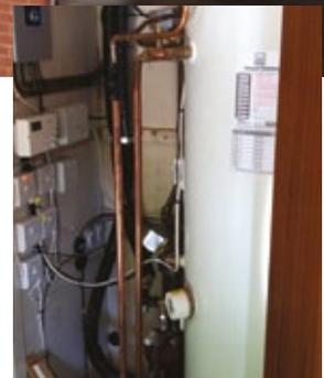
thermal panels, the wood burner or the oil fired boiler. By having a cylinder with three coils it means that each of the three heat sources can be programmed to heat the hot water independently. The oil fired boiler will only heat the water when the solar thermal and wood-burner have failed to do so.
