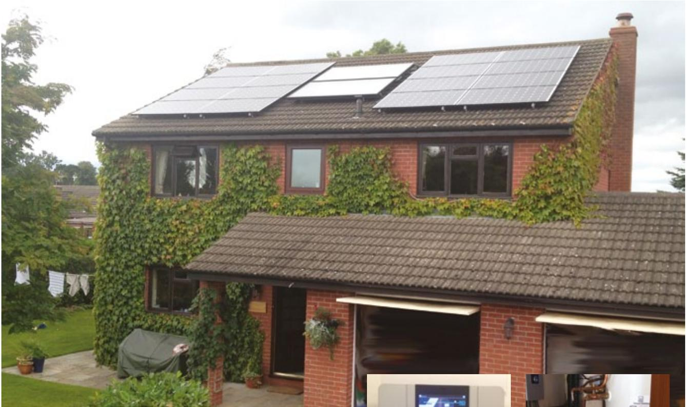
ESP Energy were asked to install two renewable systems at this property in North Shropshire. PV panels were installed to produce free electricity to the property and thermal panels were installed to produce the hot water.
